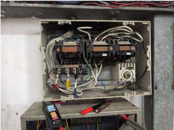
A photograph showing the interior of an open fire pump control cabinet. The cabinet is filled with various electrical components, including circuit breakers, relays, and a terminal block. Numerous white and colored wires are connected to the components. A digital multimeter and a screwdriver are placed on a metal surface in front of the cabinet, indicating a maintenance or inspection activity. | 1  |
